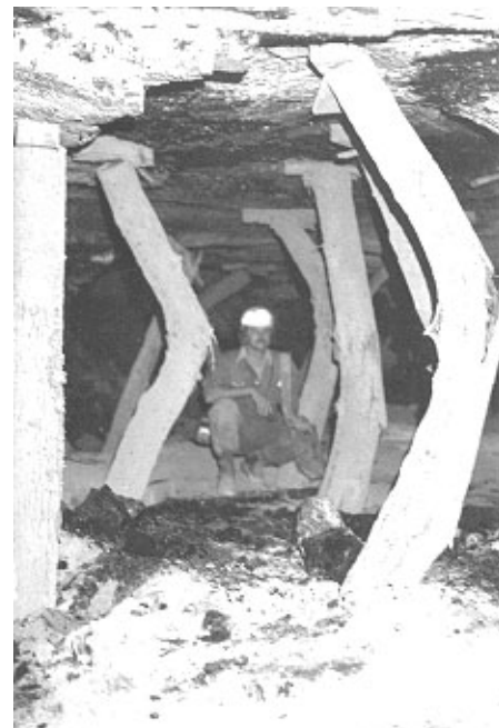
Subsidence causes supports to yield
