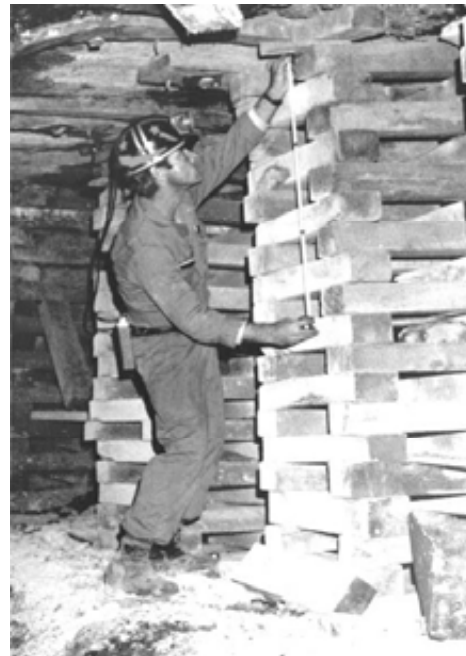
Measuring compression in support cribbing
