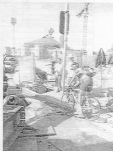
Hugh at the beginning of the construction zone.
